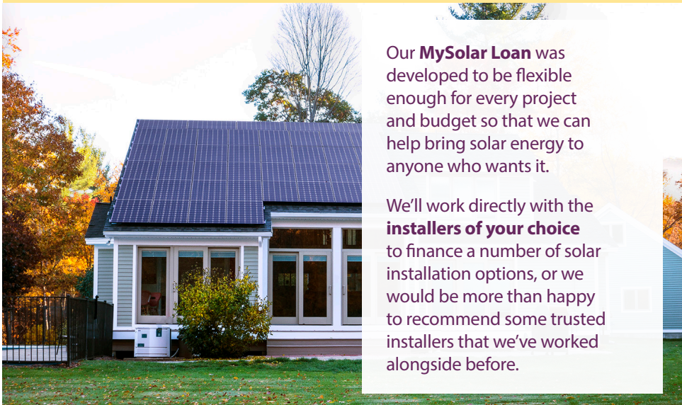
Installation photo courtesy of Northeast Solar
